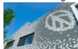
Facade Wall cladding
